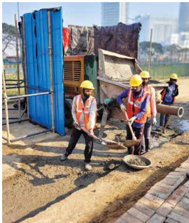
Rockwool insulation around cement mixer for noise pollution mitigation at Mahindra Luminare
